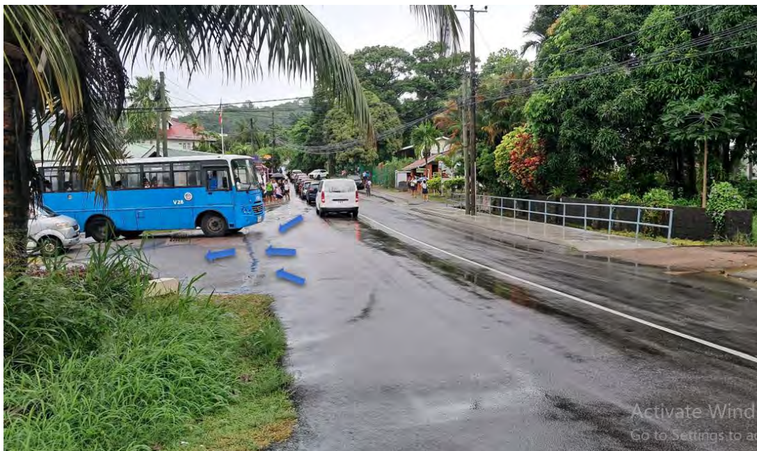
Plate 9 – Junction between main road and guest entrance to Berjaya/Aria Hotel lacks proper drainage system. As a result, flooding of and water ponding of water onto road access of Berjaya is observed (Plate 10).
